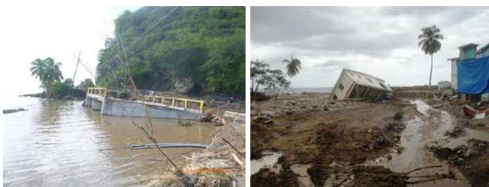
Photo 4: Damage to coastal infrastructure following tropical Storm Erika, Dominica
